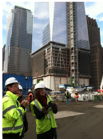
Construction at base of 1 WTC
